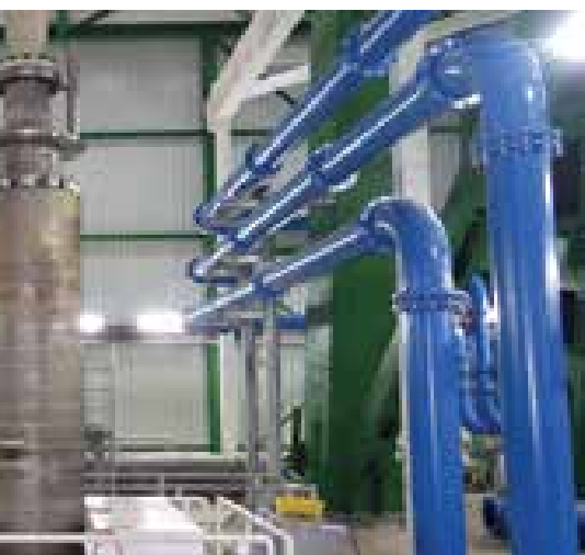
Locally ANDRITZ double-suction submersible motor pumps convey 60 million litres of water per day.
